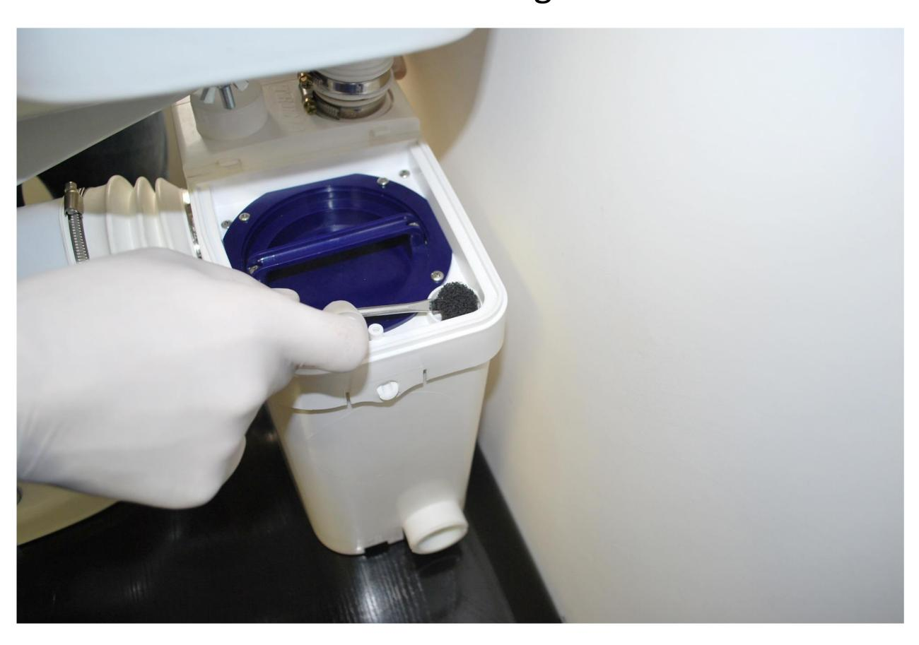
d. Clean the filter only by using air pressure (do not wet it) or change it if needed (T-PF.P116)
